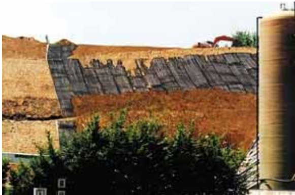
Soil filling of the TENAX MULTIMAT 110R geomats
