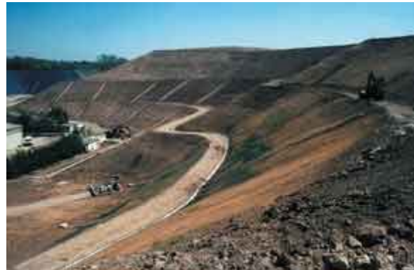
Landfill slope after geomat installation and fill soil covering
