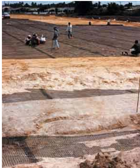
Road section on marshy soil (unconsolidated soft clay)
