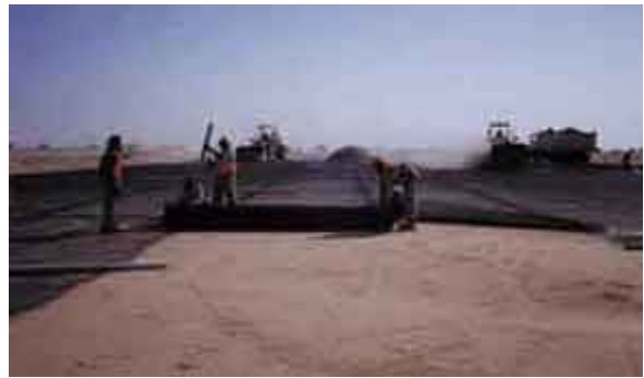
Geogrid installation by easy unrolling and overlapping
